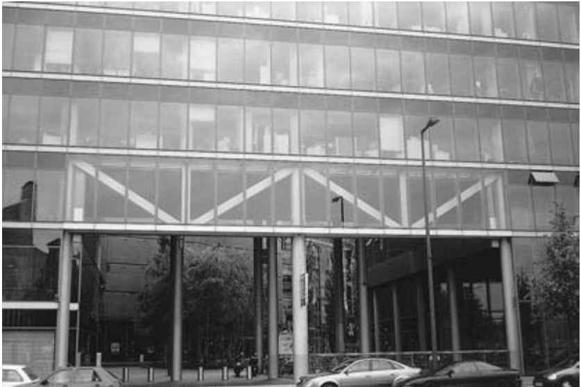
Fig. 12.5 Truss in façade, Sony Centre, Berlin.
