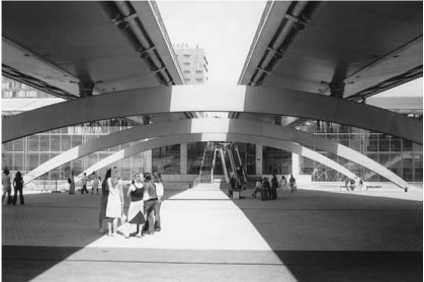
Fig. 17.4 Concrete arches supporting elevated roadway, Lille, France.
