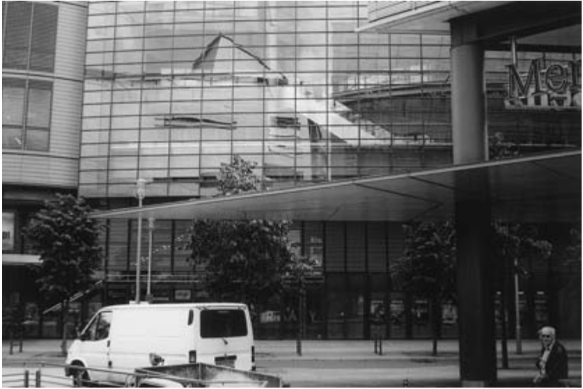
Fig. 23.1 Building with cantilevered canopy, Berlin.
