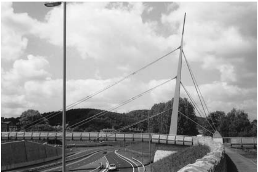
Fig. 17.3 Cable-stayed bridge, Bingley bypass, West Yorkshire.
