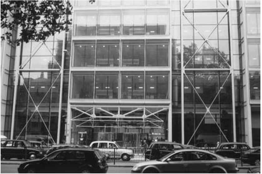
Fig. 11.8 Office building, Euston Road, London.
