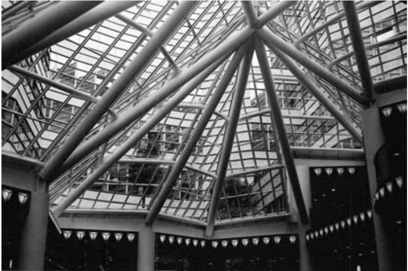
Fig. 1.2 Roof structure of Quartier 206 shopping mall, Berlin.
