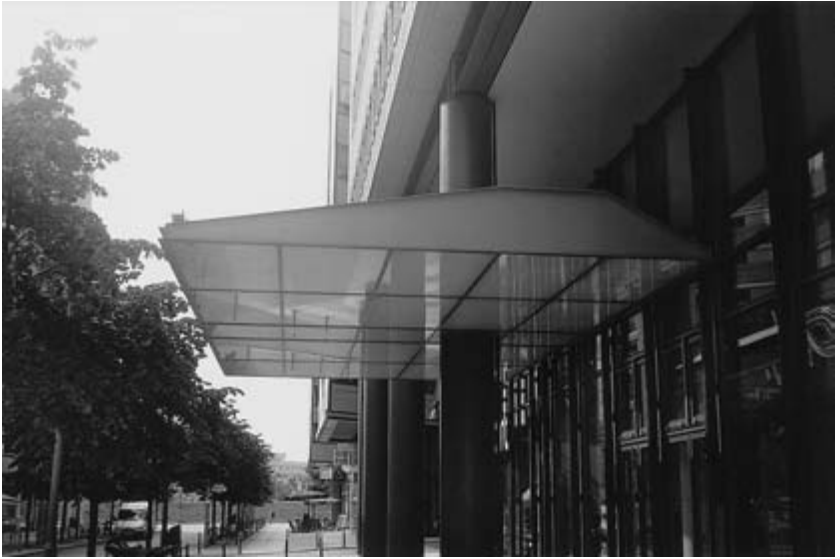
Fig. 23.2 Building with cantilevered canopy, Berlin (detail).
