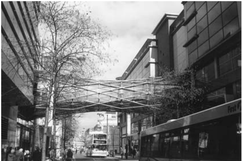
Fig. 21.2 Steel footbridge, Manchester.
