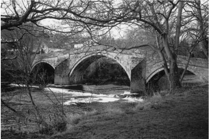
Fig. 21.1 Stone arch bridge.
