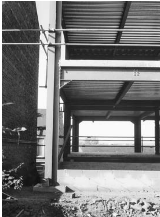
Fig. 9.2 Steel-framed building under construction.
