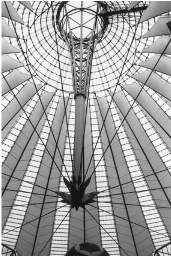
Fig. 17.1 Roof of Sony Centre, Berlin.
