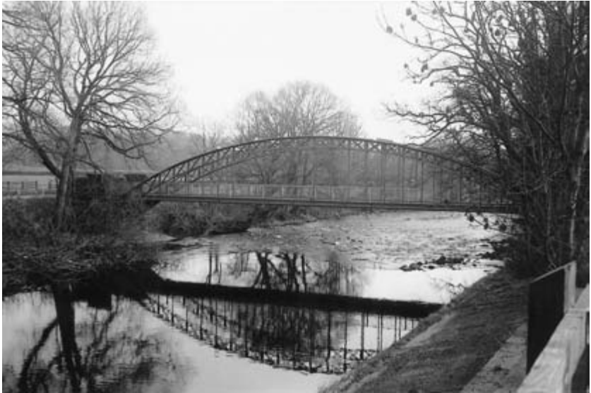
Fig. 6.1 Steel arch bridge.
