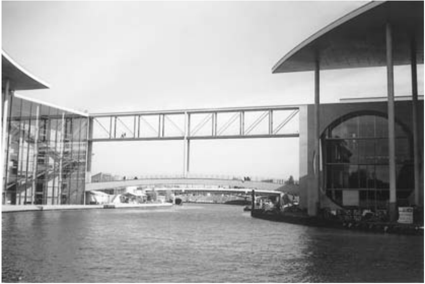
Fig. 12.4 Trussed bridge across River Spree, Berlin.
