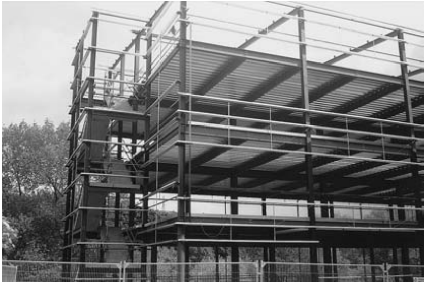
Fig. 22.1 Steel-framed office building under construction.
