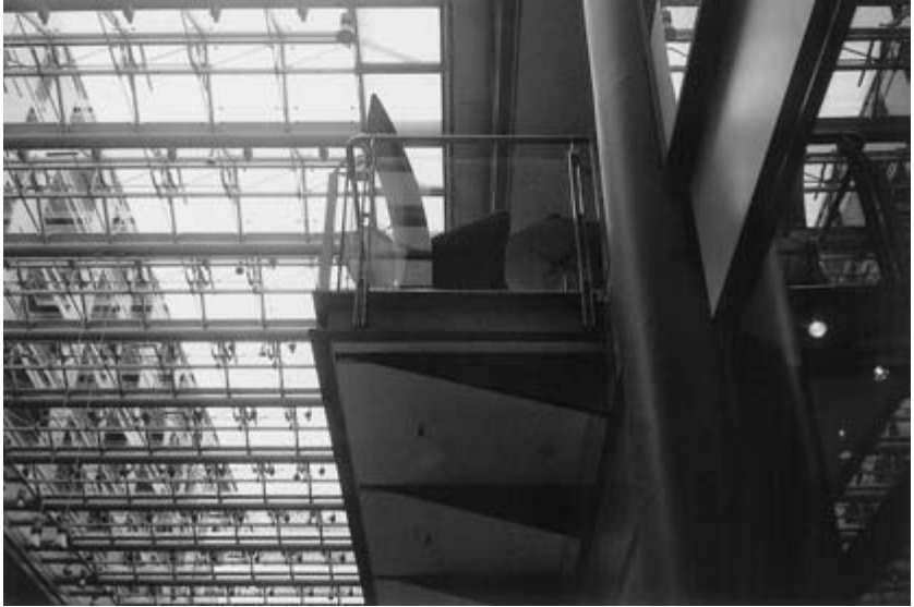
Fig. 16.25 Cantilevered balcony in shopping centre.
